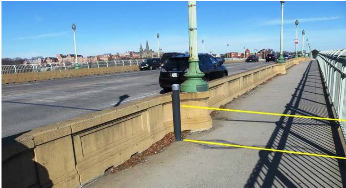
Figure 3-20. Key Bridge (Surface View)
