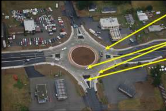
WDOT Roundabout – State of Washington, USA (Source: Flickr)
